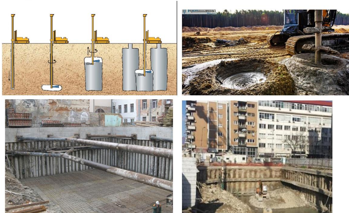
Fig.2 DSM and JG soil reinforcement applications
