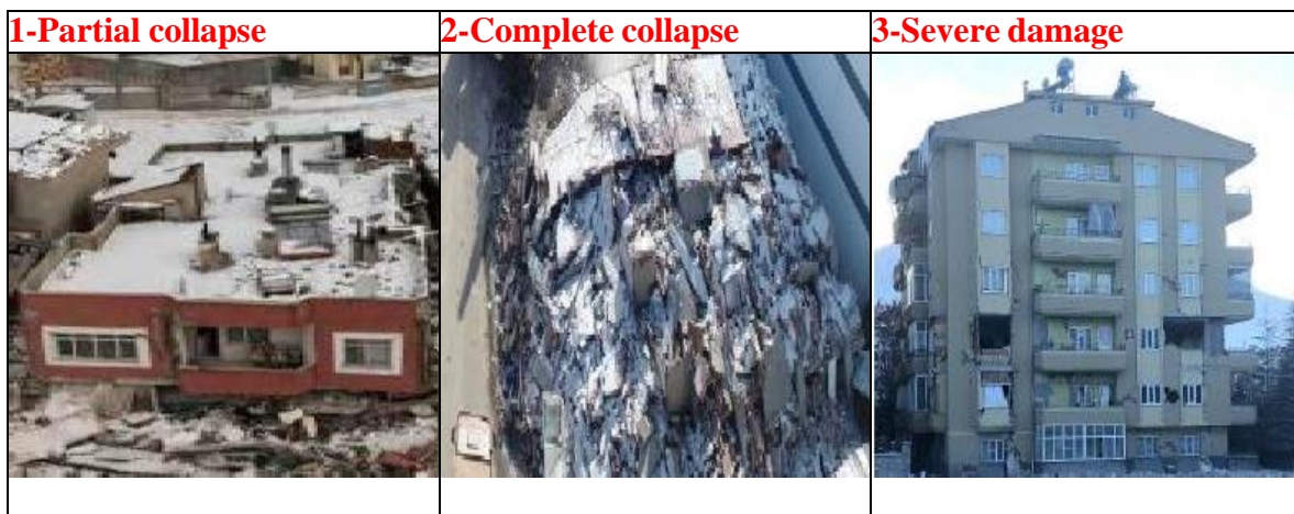
Figure 4. Damaged structures and their classifications in Elbistan
