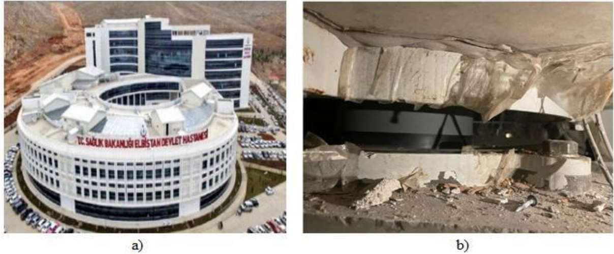
Figure 5. a) Elbistan State Hospital, b) Seismic isolator
